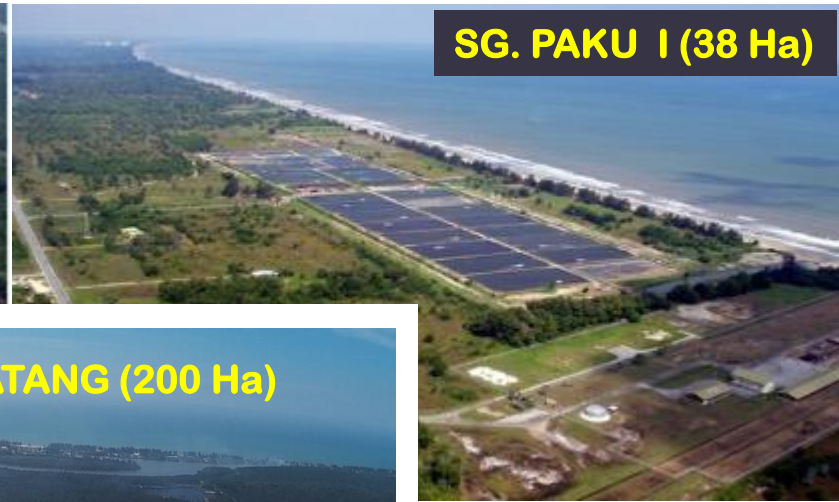
PENKALAN SIBABAU PHASE II (50Ha)
