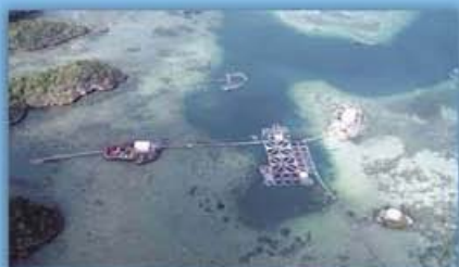
Igang Marine Substation
