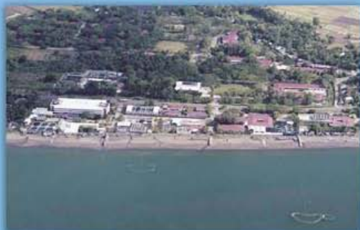
Tigbauan Main Station
