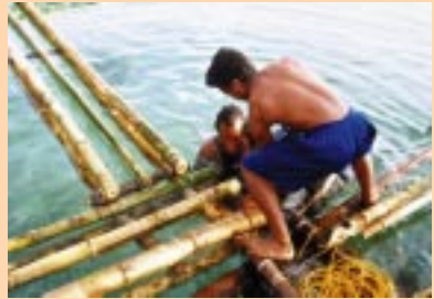
Constructing the cage
