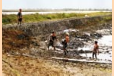
Constructing/preparing the pond
